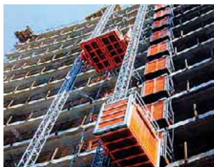
Material and working elevators
