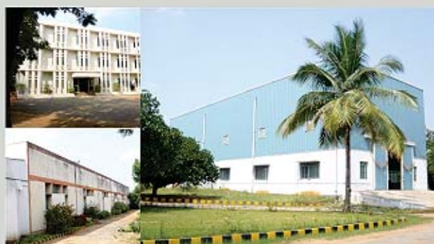
Hydraulic Cylinders & Naval Systems Plant
